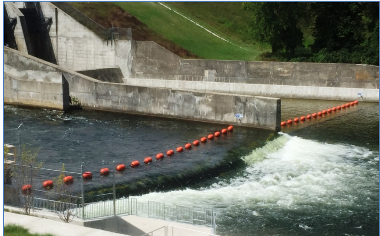
Consumers Energy installed safety buoys at Foote Dam in 2015. The energy provider continues to install buoys this summer at its hydro facilities on the Grand, Manistee, Kalamazoo and Au Sable rivers.
